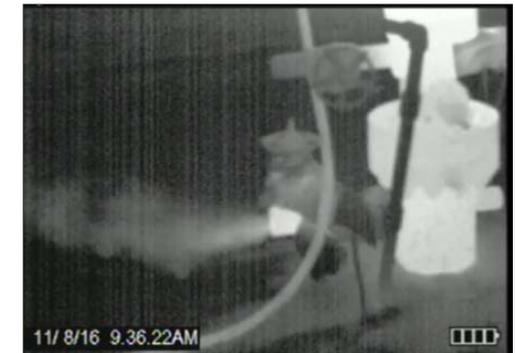
Leak from a wellhead only visible with an infrared camera
